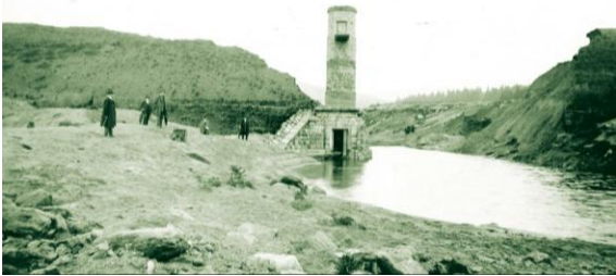
Fig. 5. View on the breach in the upstream direction, 1916 (Šámalová, 2016).
